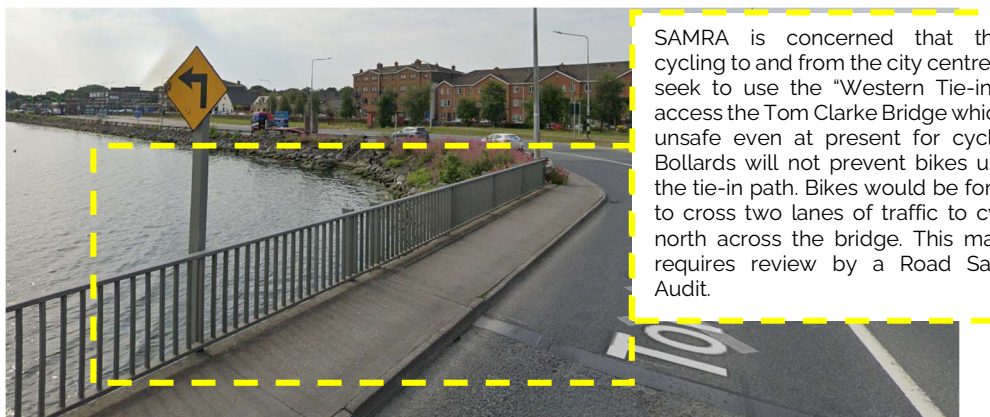
Fig. 81: Location of the "Western Tie-In" on the Tom Clarke Bridge (Source: Google Earth)
